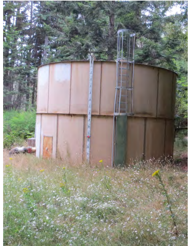
Existing Steel Tank
