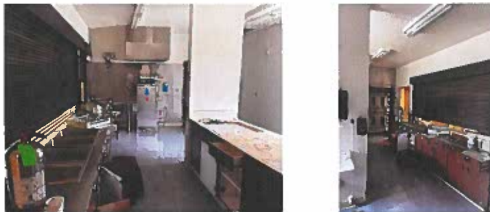
Demolition at Gymnasium - Kitchen
