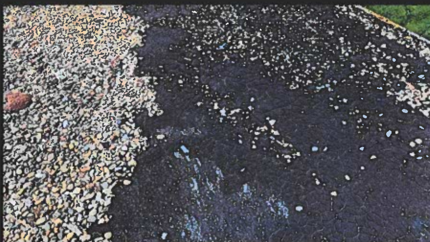
Close Up Of Roof
