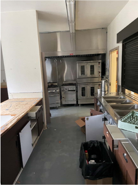
Demolition at Gymnasium
