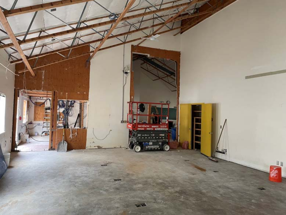
Demolition at Technical Center
