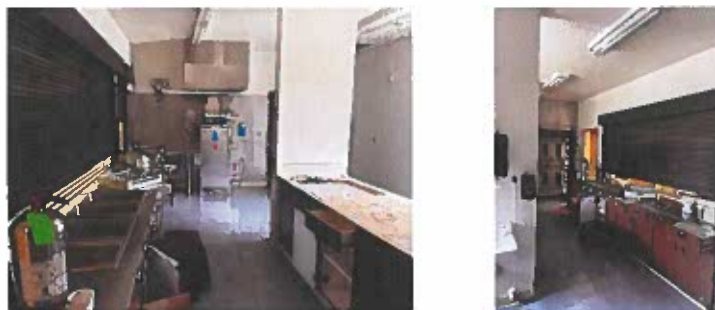
Demolition at Gymnasium - Kitchen
