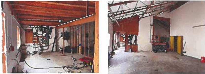
Demolition at Technical Center
