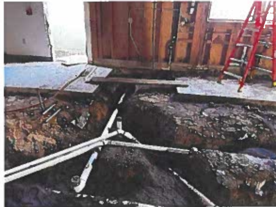
Rough-in Plumbing Gymnasium - Kitchen
