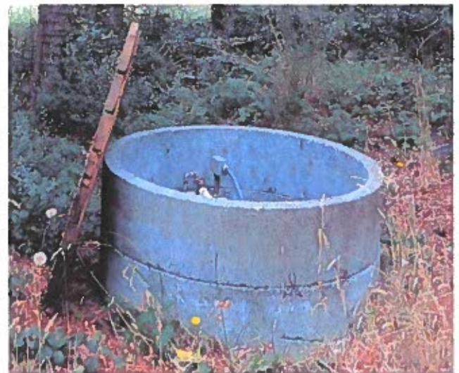
Well #2 Concrete Caisson Enclosure with Wood Lid
